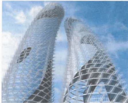
The Gullwing Twin Wind Towers
